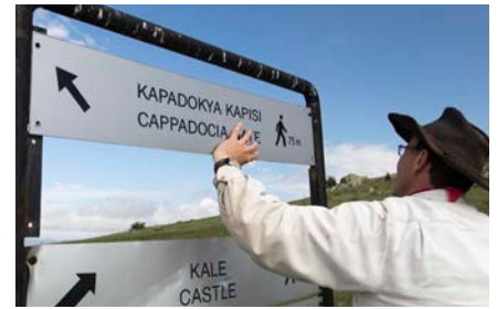
Figure 20. Repairing signs for visitors.
