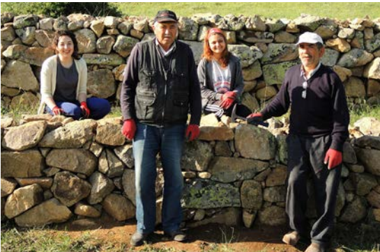
Figure 18. Architecture students from Abdullah Gül University assisted by craftsmen from Şahmuratlı village repaired stone wall reconstructions from the 2010 excavations.
