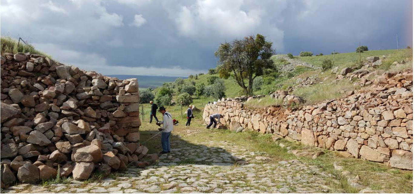
Figure 16. Clearing the Cappadocia Gate of vegetation with students from Abdullah Gül University for photogrammetric modeling.
