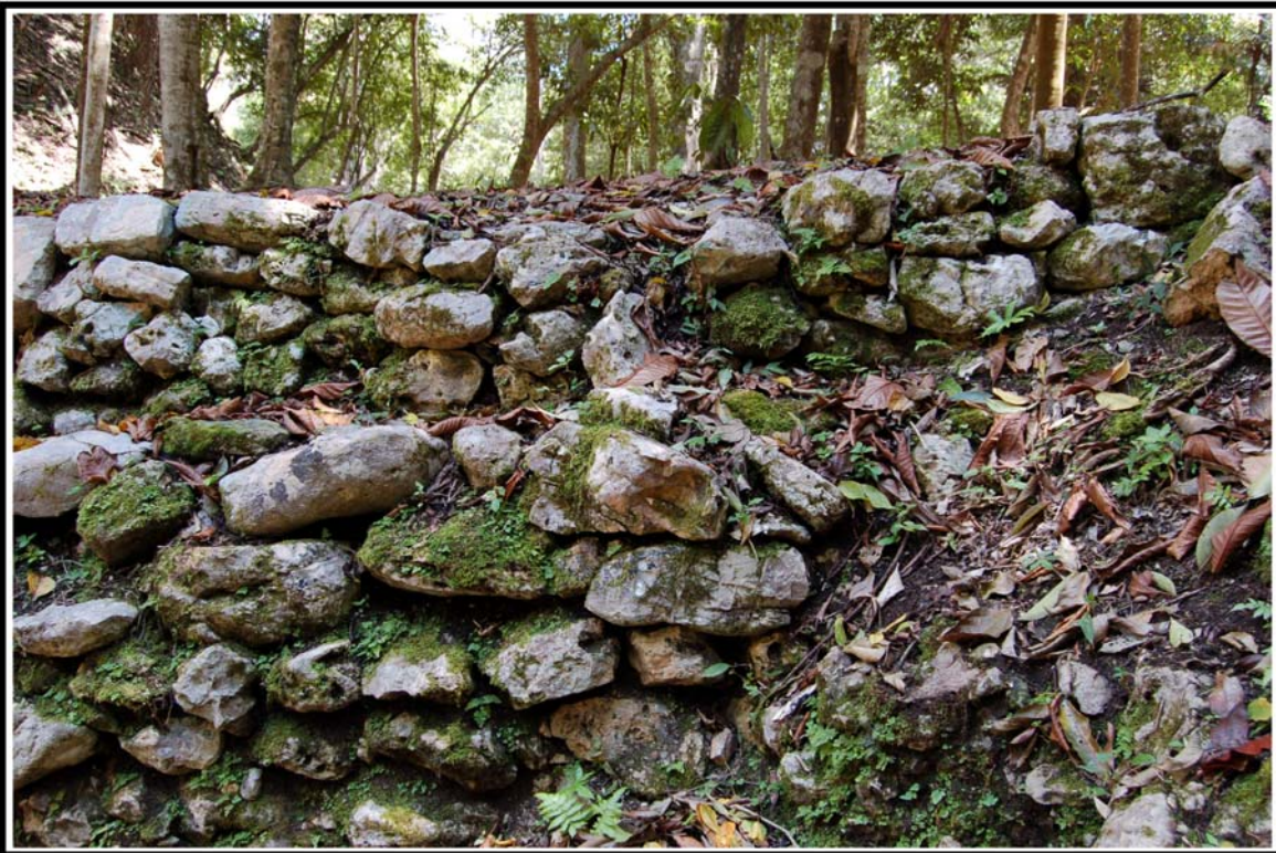
Figure 14: The cut stone lining of Reservoir B
