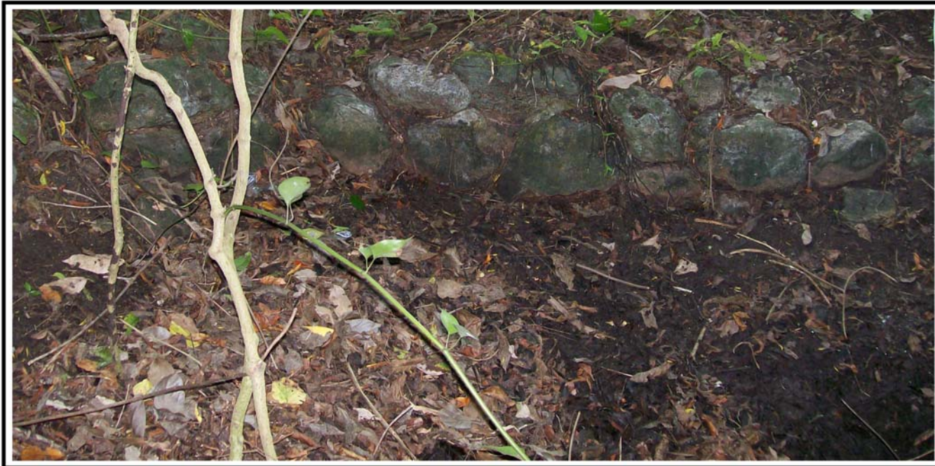
Figure 11: Wall lining of the A18 Reservoir. Photo Courtesy of Andrea Slusser
