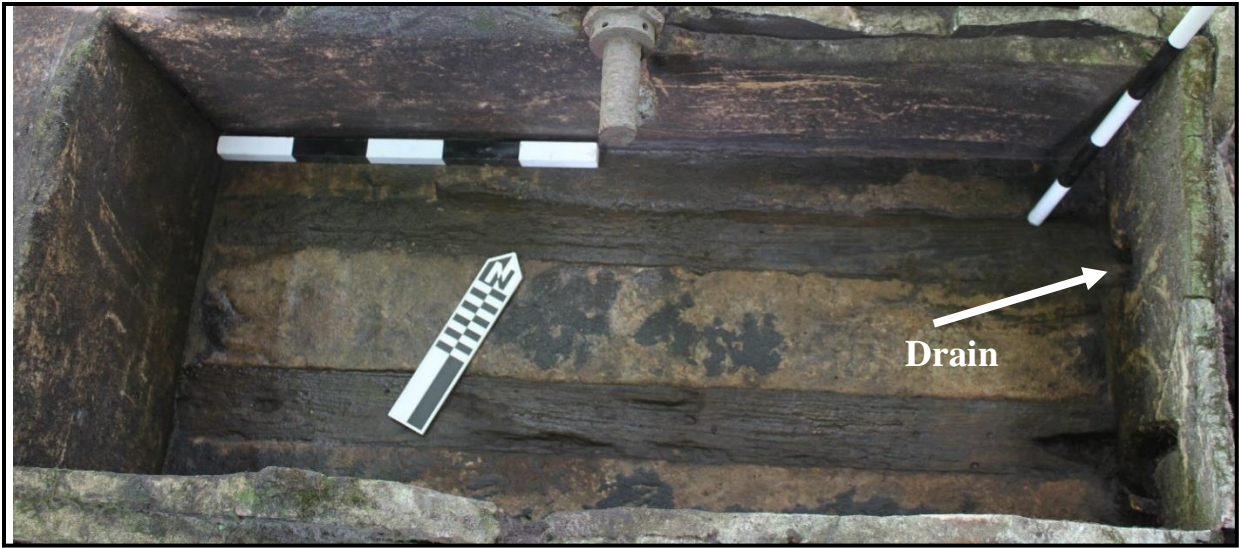
Figure 43. Floor of gear box. Wood inserts are visible and run parallel to each other. One wood plank seems to line up with a drain hole in the east wall of the box. Reason for wood panels is unknown though given the alignment with the gear attachment arms it may have been related to the gear placement.
