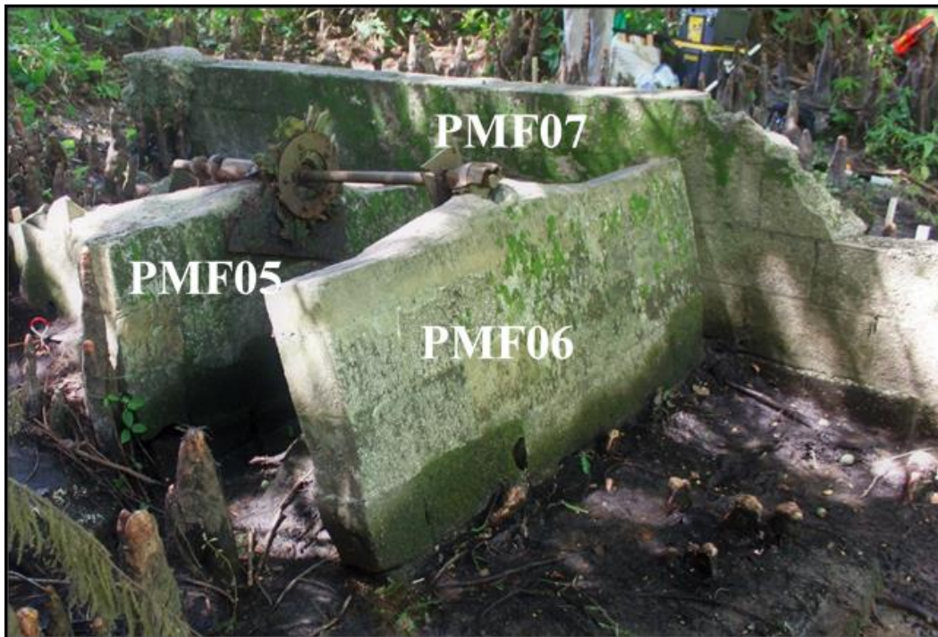
Figure 23. Existing mill foundation, walls are labeled with their feature numbers.
