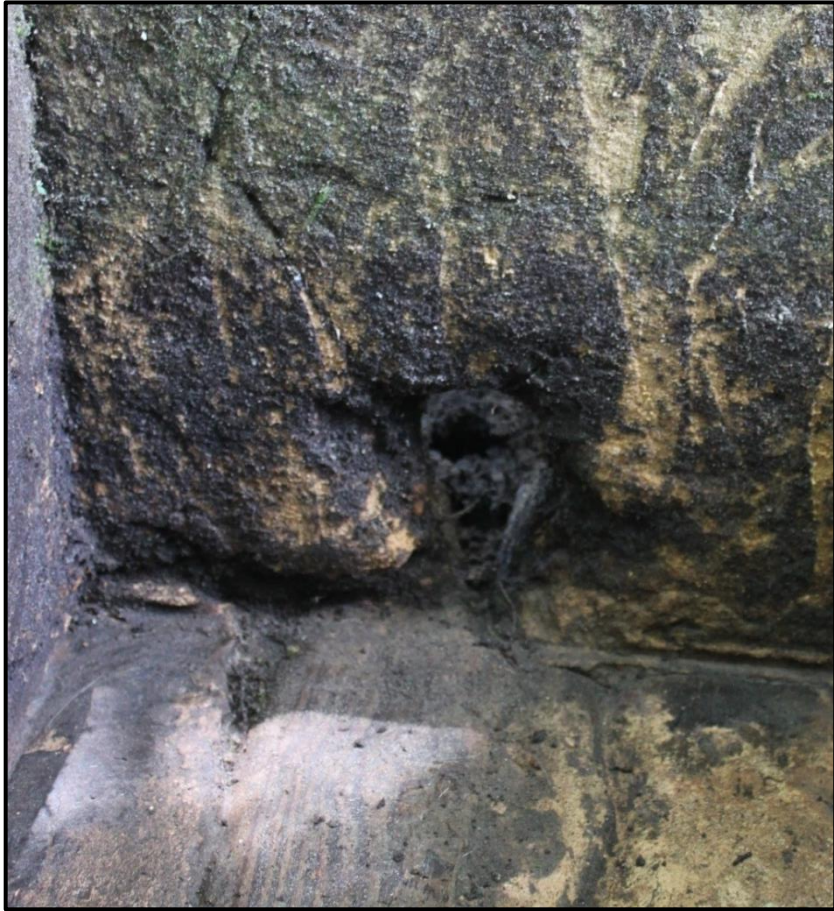
Figure 44. Drain hole in the eastern wall of the gear box.
