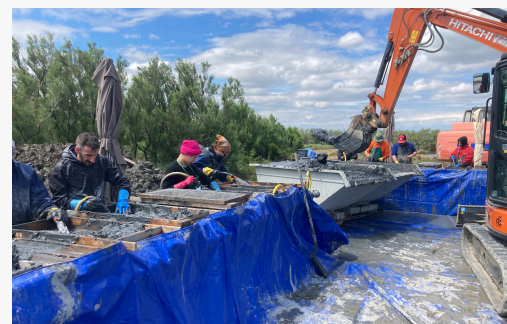
Water screening of excavated sediments during recovery operations.
