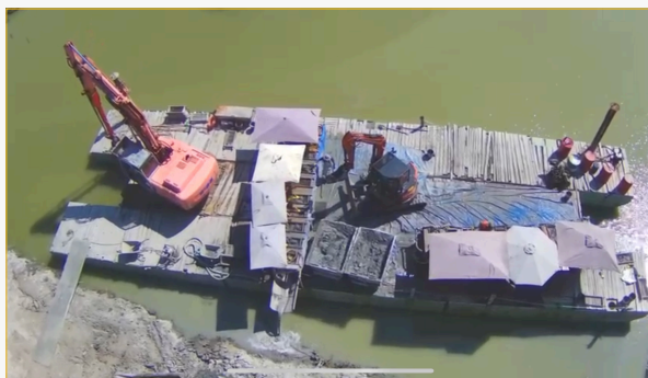
Barge-based excavation during a submerged recovery mission.
