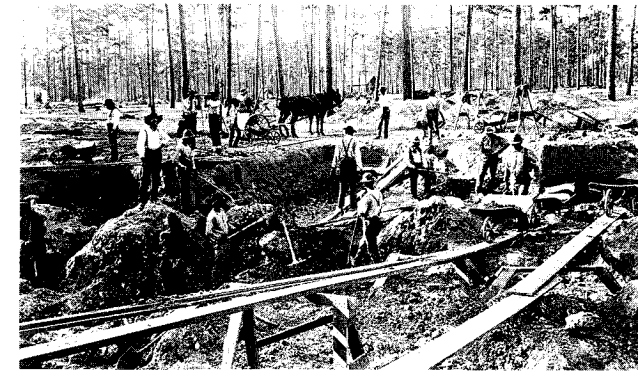
FIGURE 10. Phosphate mining in pine flatwoods near Bartow, Florida circa 1900. (Courtesy of Florida Institute of Phosphate Research.)
