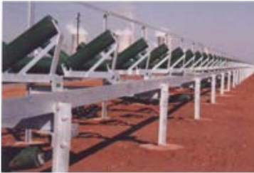
Support structure in the ground with steel beams with U or tubular cross section
